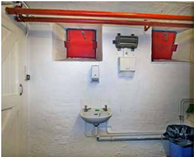
The 'Oben' blast valves in the male toilets
